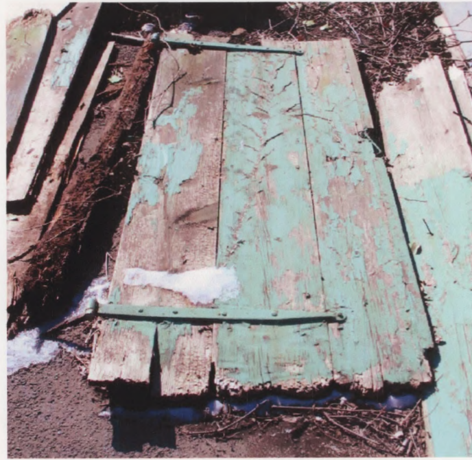
19TH-CENTURY DOOR FROM SOUTH WALL WITH ROTTED STUD ATTACHED
