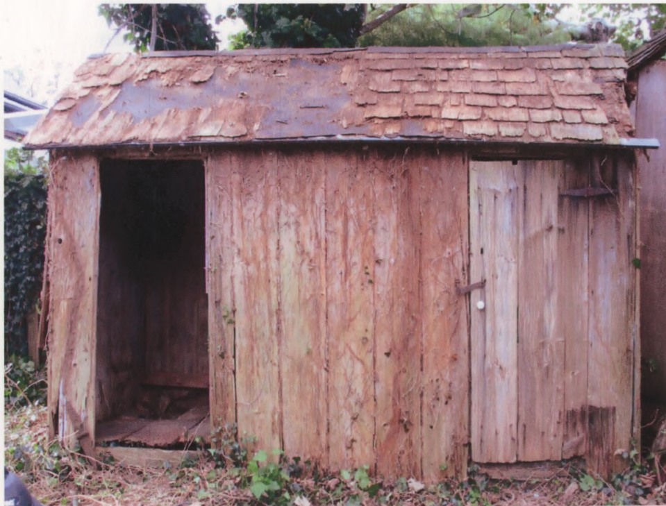
BATH HOUSE, EAST WALL
