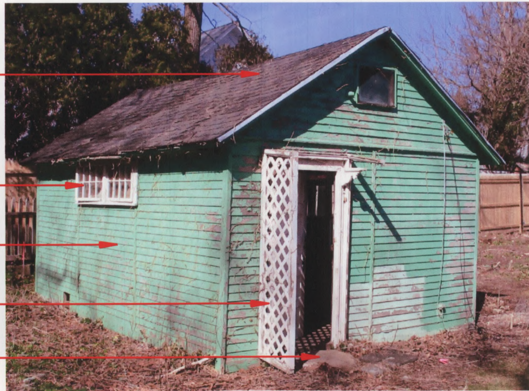
THREE ORIGINAL CLAPBOARD WALL PANELS, 6' WIDE, WITH BATTENS COVERING THE JOINTS
