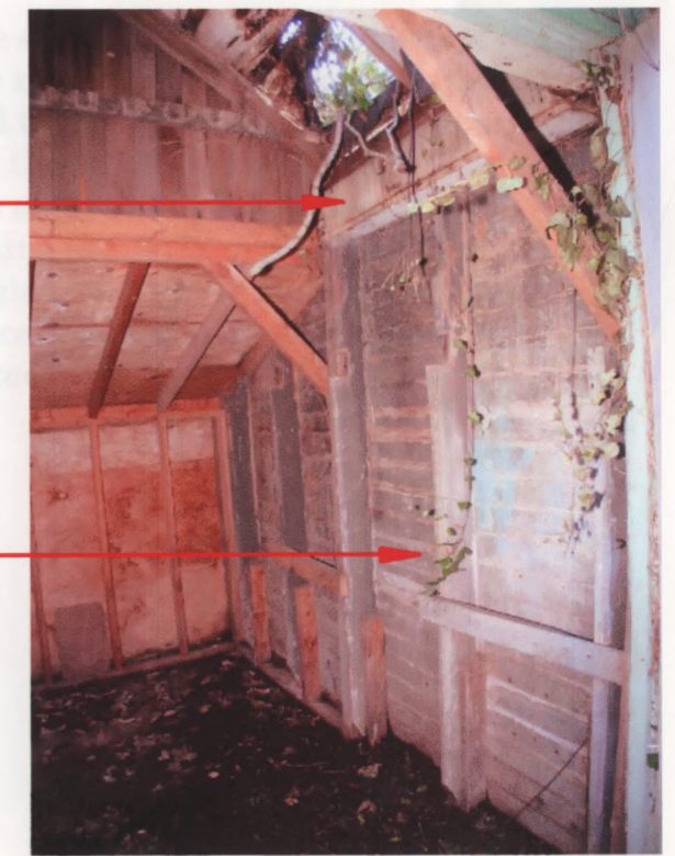
BOAT HOUSE, INTERIOR VIEW OF WEST AND NORTH WALLS
