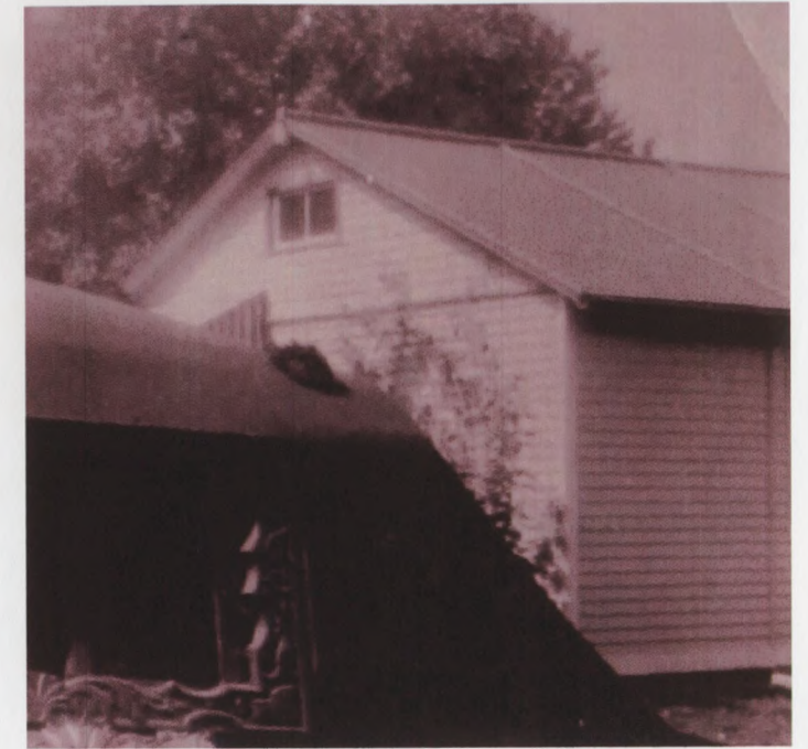
DETAIL OF UNDATED PHOTOGRAPH SHOWING THE GREEN CLAPBOARD ROOF PANELS, RIDGE ROLL AND STRIPED AWNING OVER THE DOOR.
