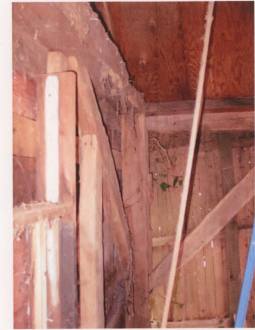
INTERIOR VIEW SHOWING HEWN OAK FRAME OF THE ORIGINAL BUILDING: THE NORTHWEST CORNER POST, SOUTH PLATE, WEST TIE BEAM AND WIND BRACES
