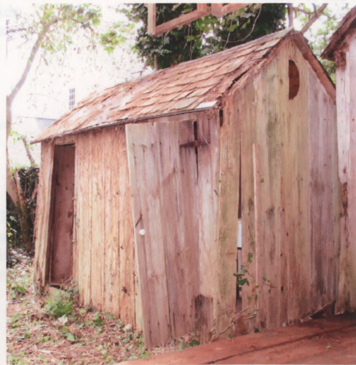
BATH HOUSE, EAST WALL AND NORTH WALL
