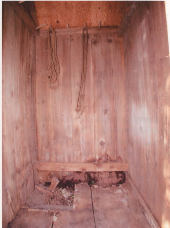
INTERIOR OF SMALLER SOUTH ROOM SHOWING PEGS SET IN THE PLATE AND GABLE TIE
