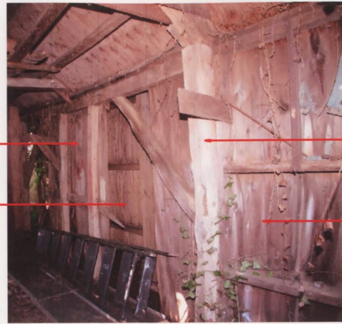
NORTH WALL FROM INTERIOR
